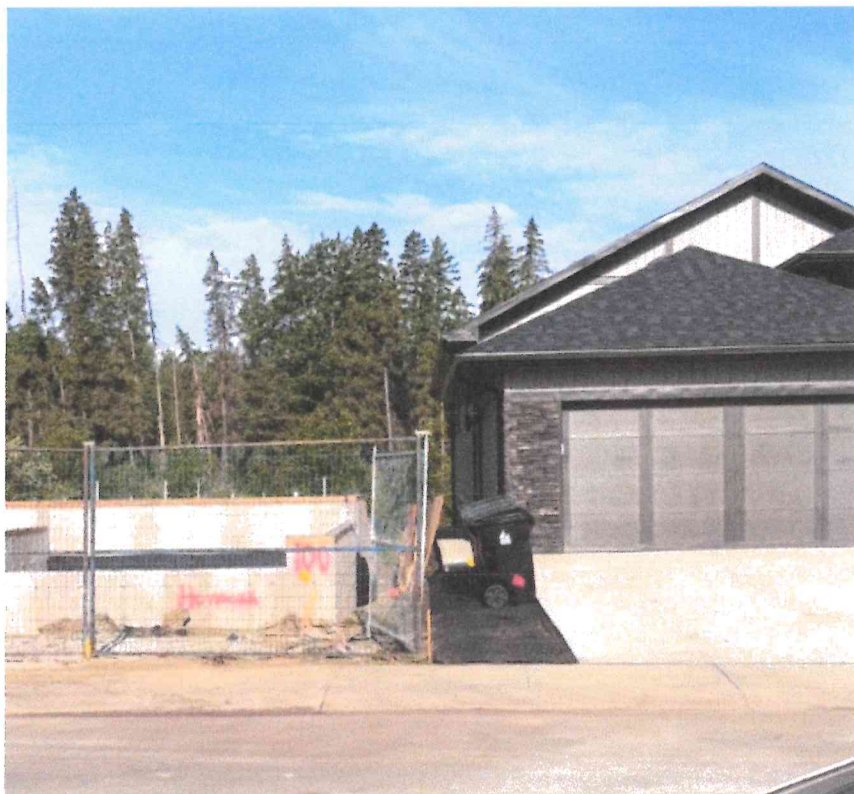
No space between homes at 100 Hemingway Crescent.
