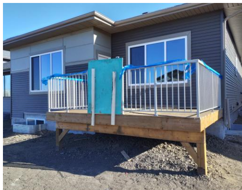
Site photo showing as-built rear uncovered deck, measuring 1.27 m in height and 3.37 m by 4.40 m in size
